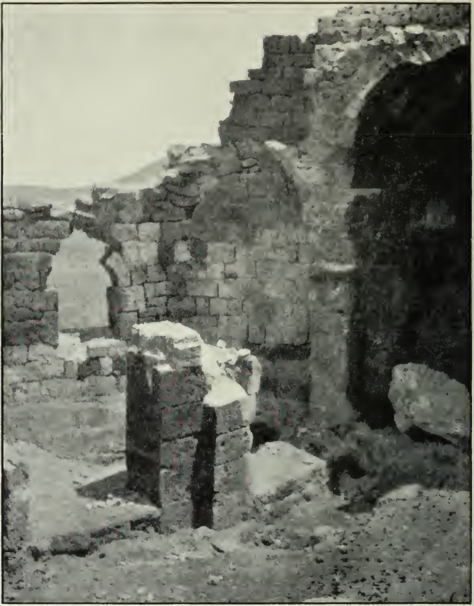
FIG. 68.—No. 10, interior from S.-W.
